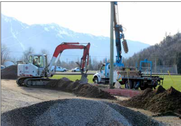
Construction work replacing sewer pipes continues on Seabird Island
