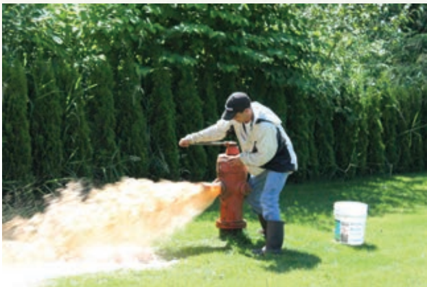
John flushing the Seabird water system
