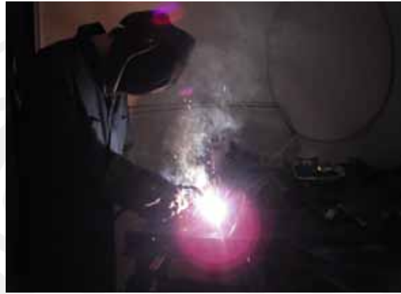
Josh LaCroix welding the frame for the new stage.
