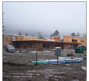
High School Construction
