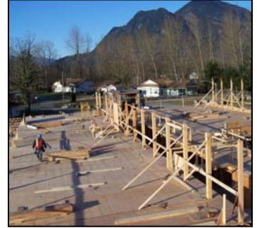
High School Construction
