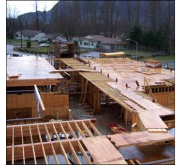
High School Construction
