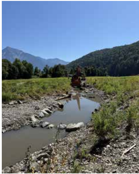
During construction, the added rocks to hold water in the channel and logs can be seen better while the water was low in the construction phase.
