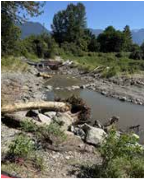
During construction, the added rocks to hold water in the channel and logs can be seen better while the water was low in the construction phase.
