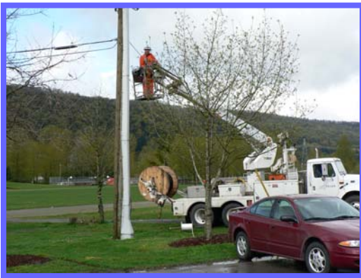
TELUS installing cable for wireless network
