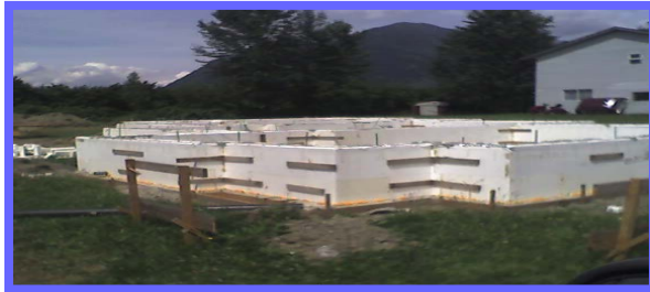
New Insulated Concrete forms
