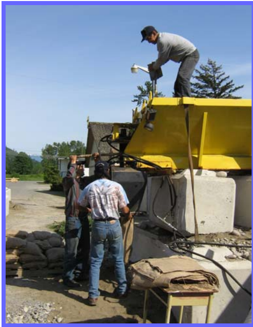
Sandbagging in case of flood
